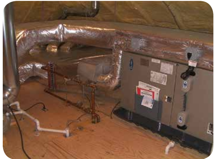
Carrier 5-ton A/H with same options as 1 st floor systems.
