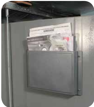
Anodized (as paint primer) and painted aluminum instruction holder – no zone legend is needed on the 3 single-zone A/Hs. My bronze company plaque can be seen just right of the Carrier logo (center image).
