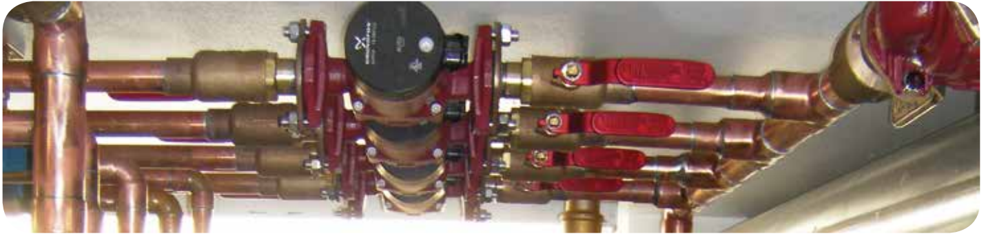
Grundfos Alpha circulators were chosen to maximize performance with the lowest electricity consumption.
