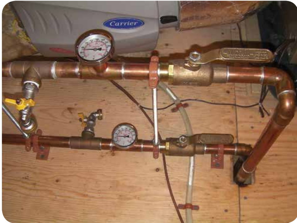
Lacquered bronze handles designate "Heating Supply" and "Heating Return" lines to the hot water coil associated with the attic A/H.
