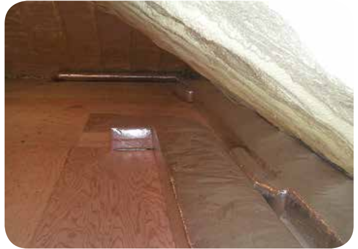
The supply trunk on the right replaced 3 excessively long flex run-outs.
