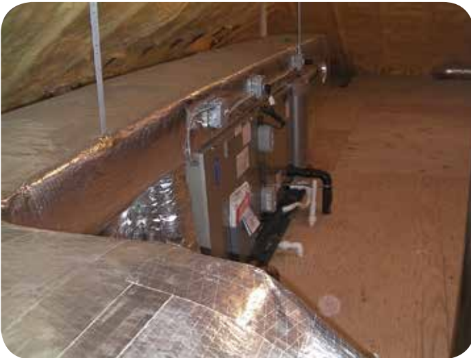
Carrier 5-ton A/H with same options as 1 st floor systems.
