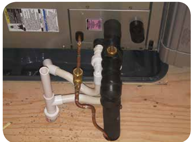
Valves on refrigerant lines and unions on condensate drains facilitate future maintenance.
