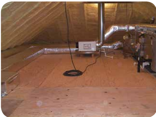
The space is now accessible without stepping on ducts, or mis-stepping on unfastened plywood, through the insulation and sheetrock ceiling below.
