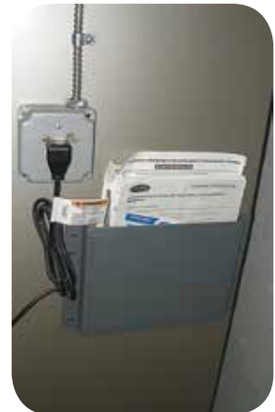
Anodized (as paint primer) and painted aluminum instruction holder – no zone legend is needed on the 3 single-zone A/Hs. My bronze company plaque can be seen just right of the Carrier logo (center image).
