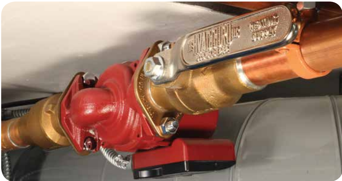
Nickel-plated bronze "Heating Supply" handles on 1-½" valves that isolate the supply line to the Triangle Tube indirect-fired water heater.
