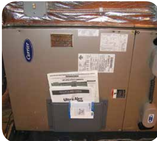
Anodized (as paint primer) and painted aluminum instruction holder – no zone legend is needed on the 3 single-zone A/Hs. My bronze company plaque can be seen just right of the Carrier logo (center image).
