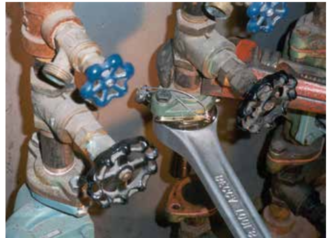
Figure 24: The valves I invented replace this conglomeration of fittings, gate valves and problematic flanges.
